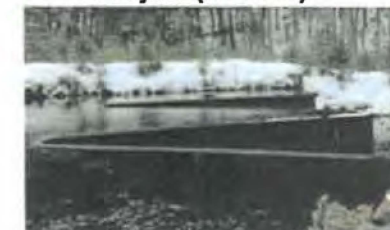
Stone Creek Hydro Project (12 MW)
