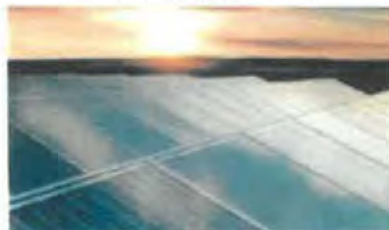
White Bluffs Solar Station (38 KW)
