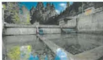
Packwood Lake Hydro Project (27 MW)
