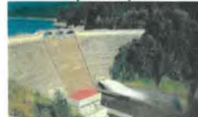
Portland Hydroelectric Project (37.5 MW)
