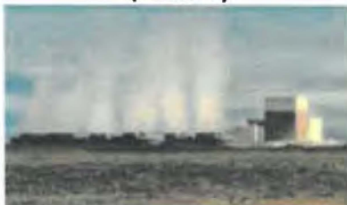
Columbia Generating Station (1,207 MW)
